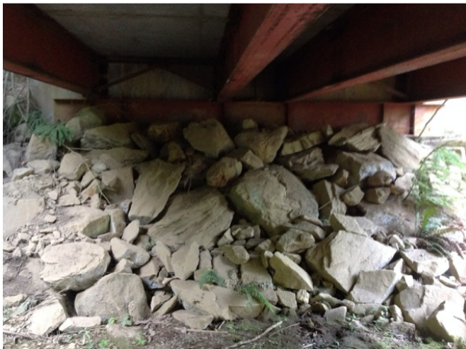
Left Bank Abutment when facing downstream
