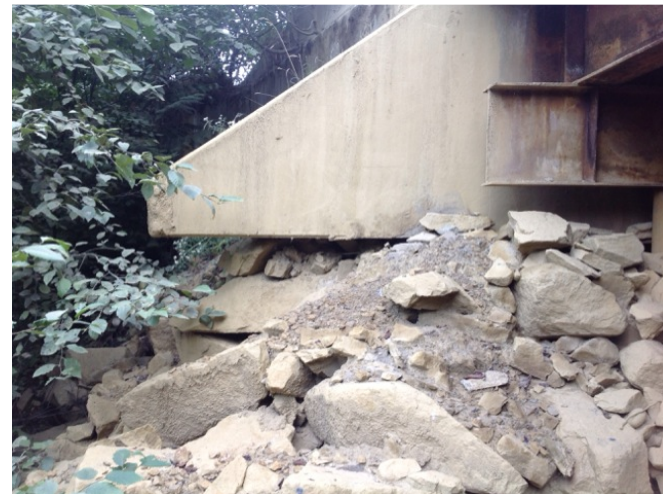
right downstream ballast wall
