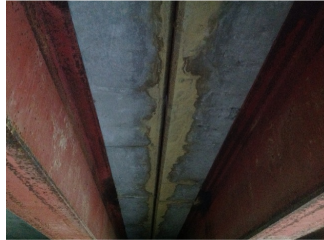
differing depths of deck panels
