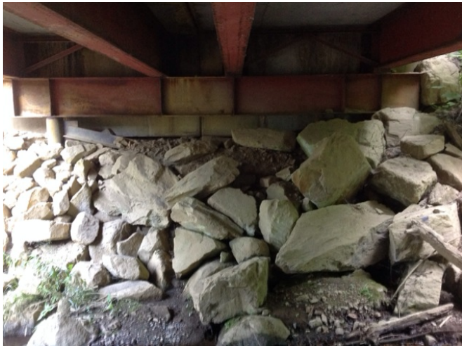
Right Bank Abutment when facing downstream
